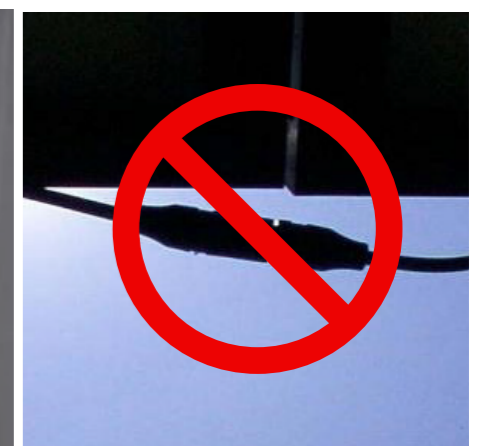
Example of improper cable installation 15
