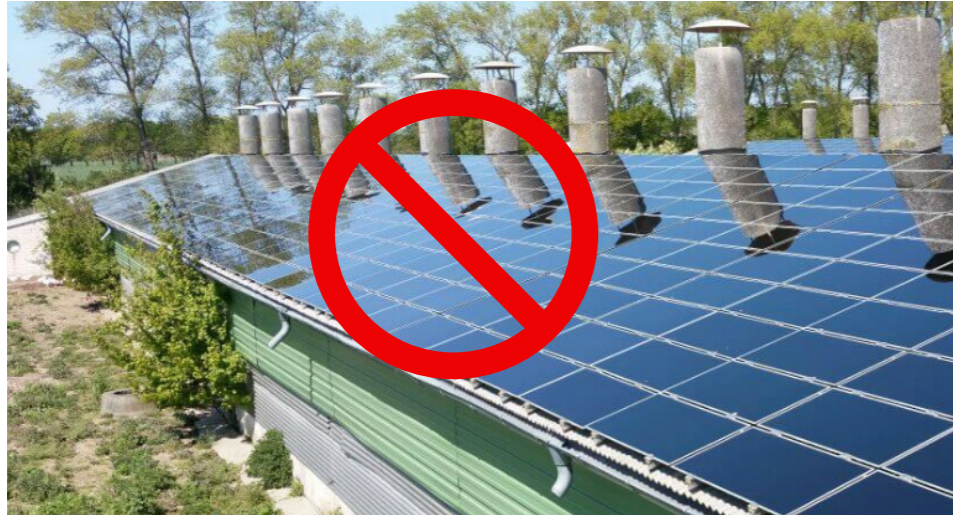
Example of risk of accumulation of deposits on the glass surfaces of the panels due to proximity to exhaust stacks 6
