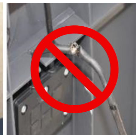
Example of improper cable installation 16
