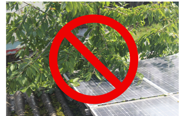
Growing plants lead to shadows on the cells: Hot spot risk, loss of performance 3
