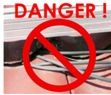
Improper cable installation 13
